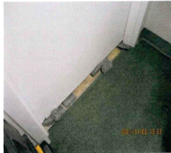
Photo 24. Steel Wool Placed Under Door
