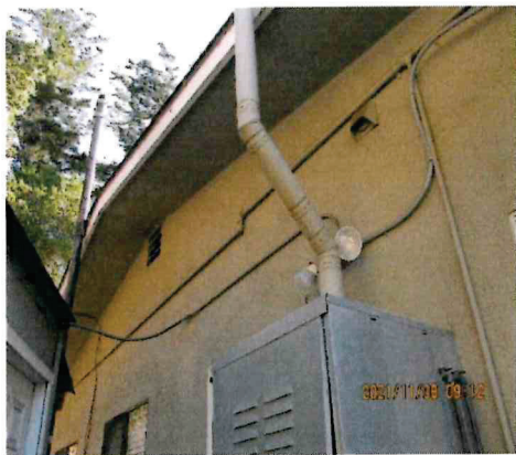
Photo 17. Gas Line Runs on side of building to DWH
