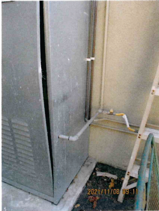
Photo 19. Non-compliant Gas connection
