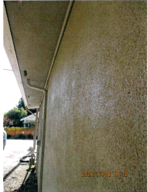
Photo 16. Gas Line Installed below Roof overhang
