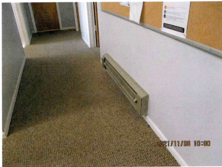
Photo 31. Example of Interior Non-operable Wall-mount Baseboard Heaters
