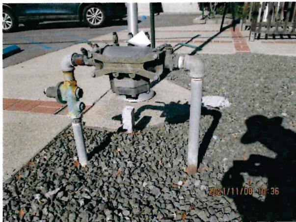
Photo 21. Domestic Water Backflow Preventer
