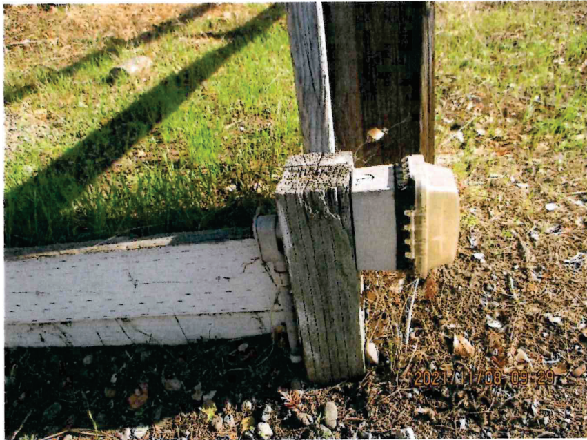
Photo 30. Non-compliant Exterior Convenience Outlet
