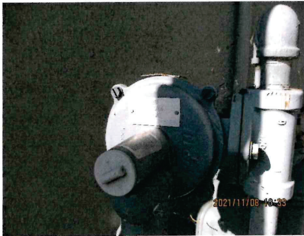
Photo 15. Gas Service Regulator
